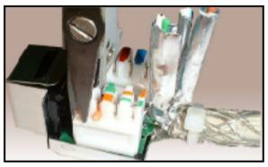
6. Arrange the wires according to the color and use punch down tool terminate each pair.)
