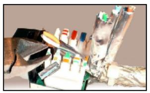
5. Cut each single wire's aluminum foil off subject to terminated IDC position length.
